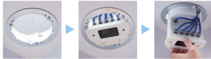
(設置・取付の様子)
